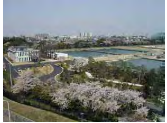
Photo: Oldest water treatment plant in Japan using the slow sand filtration method (Tokyo, Sakai Purification Plant) Treated volume: 315,000m 3 /day
