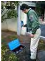
Leakage survey by private company
