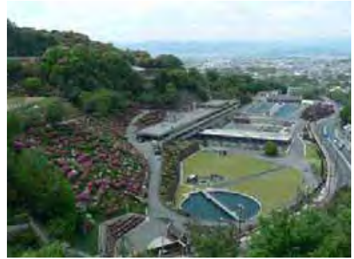
Photo: Oldest water treatment plant in Japan using the rapid sand filtration method (Kyoto, Keage Treatment Plant) *This water treatment plant was constructed in 1912. Treated volume: 99,000m 3 /day
