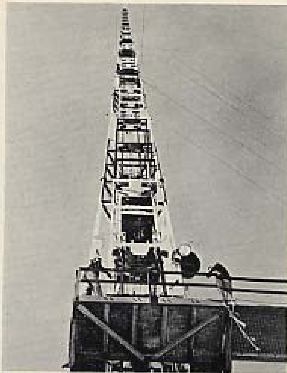
Fig. 9. The Health Physics Research Reactor Mounted on Hoist Car on Bren Tower
