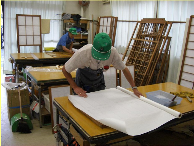
Replacement of paper on sliding doors and screens
