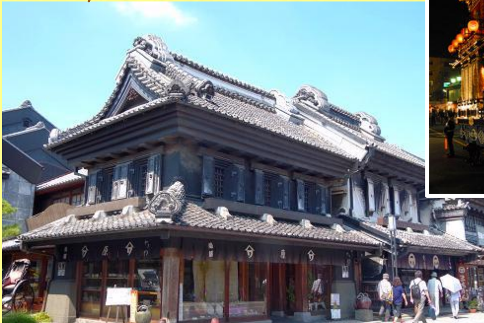
Townscape of Kura Storehouse
