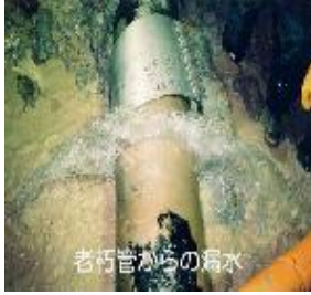
Example of dilapidated facility
