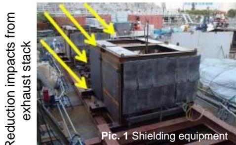
• A 16 mm thick steel plate (shielding effectiveness: 50%)
