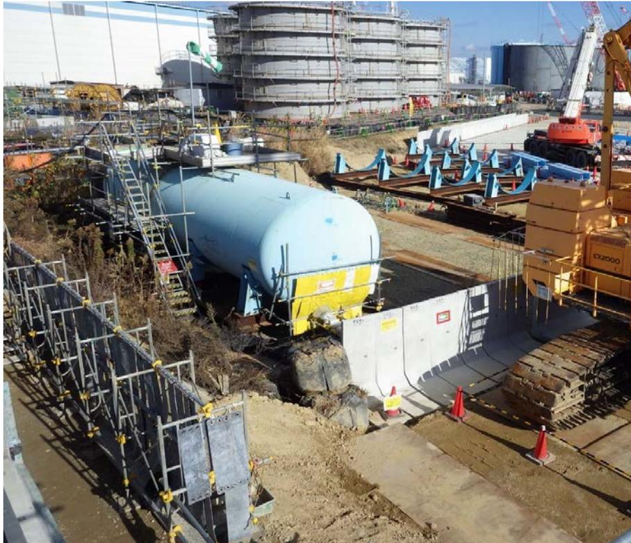
The L-shaped concrete retaining walls used during the contaminated tank disassembly work and the lead plate shielding partitions
