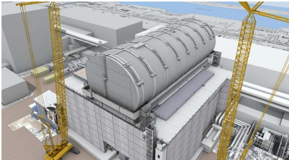
1F-Unit 3 Reactor Building 5F Conceptual Illustration of the Fuel Removal Framework as
