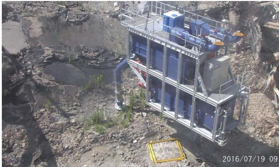
1F - Unit 1 Reactor Building 5F Suction of rubble pieces such as roof blocks using large rubble suction machine
