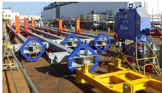
▲ Basic assembly of nozzle unit steel frames
