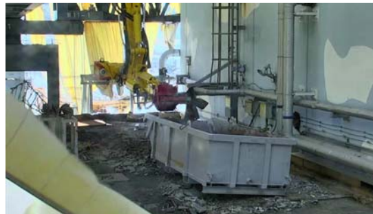
▲ Removal using small grippers
