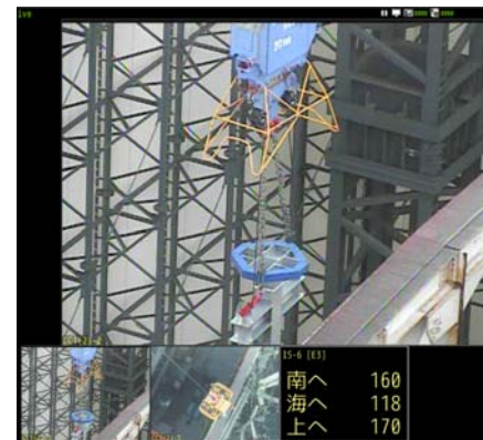
▲ Installation of nozzle unit steel frame using remote guidance system
