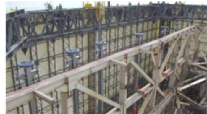
▲ Nozzle unit steel frame installation (East side) (East side 7 locations, west side 6 locations)
