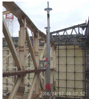
▲ Installation of nozzle unit steel frame using remote guidance system
