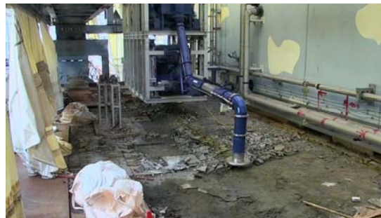
▲ Suction using rubble suction machine
