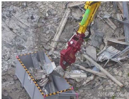
▲ Obstacle removal using small grippers (moving)
