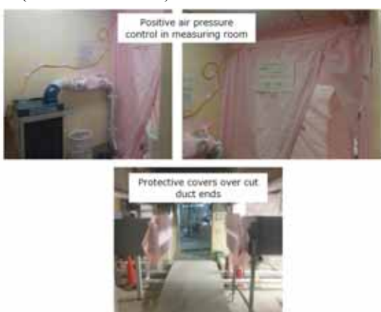
Contamination control during expansion work
