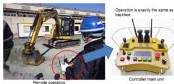
Backhoe equipped with robot
