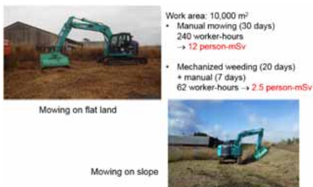
Mechanization of mowing work
