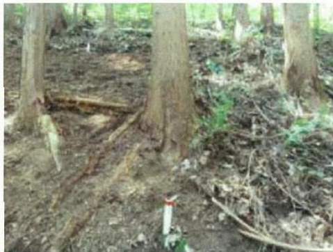
Photo 4. Conditions before and after removing fallen leaves, etc. (The right side of the photo shows the condition before removal. The left side shows the condition after fallen leaves, etc., were removed.)
