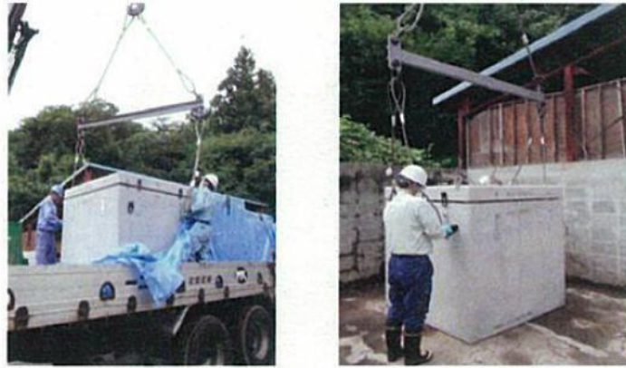
Photo 1: Positioning of a concrete container
