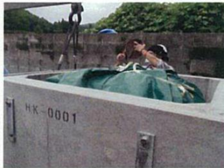
Photo 2: Placing the flexible container bag in the concrete container.
