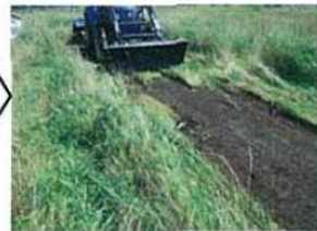
A front loader was used, the grass was torn up and removed.
