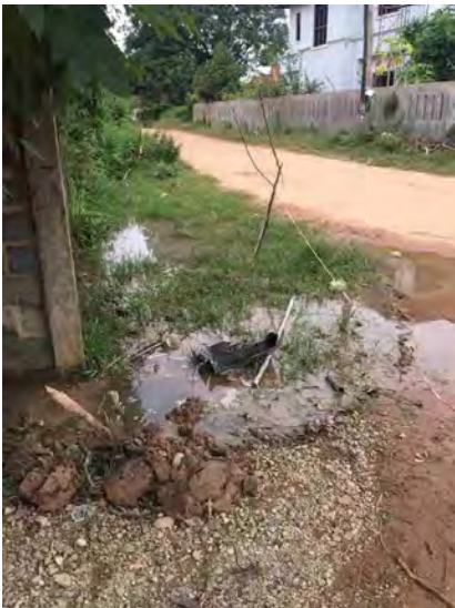
Water Leakage (Photo: NPNL)
