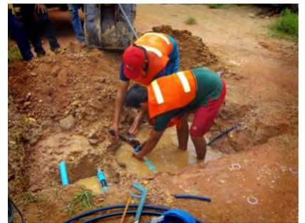
Water Leakage (Photo: NPNL)
