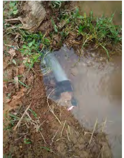
Water Leakage (Photo: NPNL)
