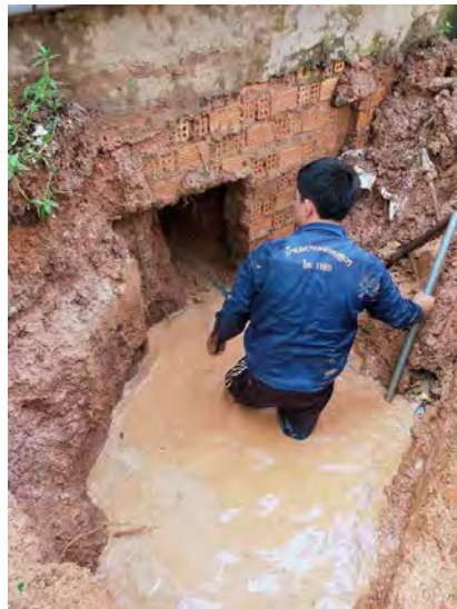
Water Leakage (Photo: NPNL)
