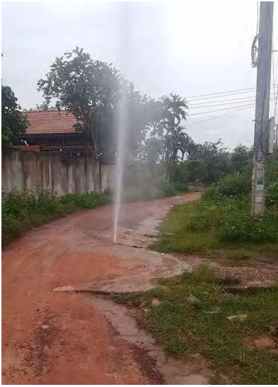
Water Leakage (Photo: NPNL)
