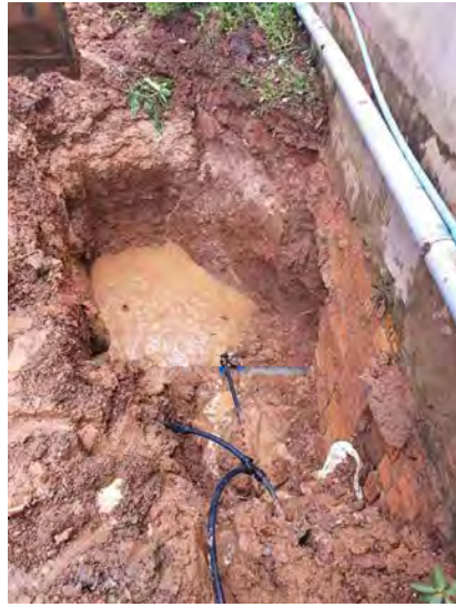
Water Leakage (Photo: NPNL)
