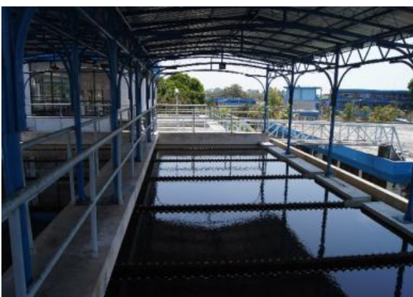
No.15 Sedimentation Tank in Brushn Water Treatment Plant
