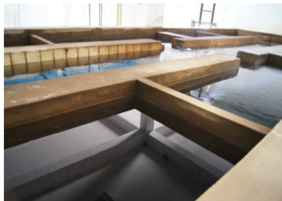
No.16 Filtration Tank in Brussels Water Treatment Plant
