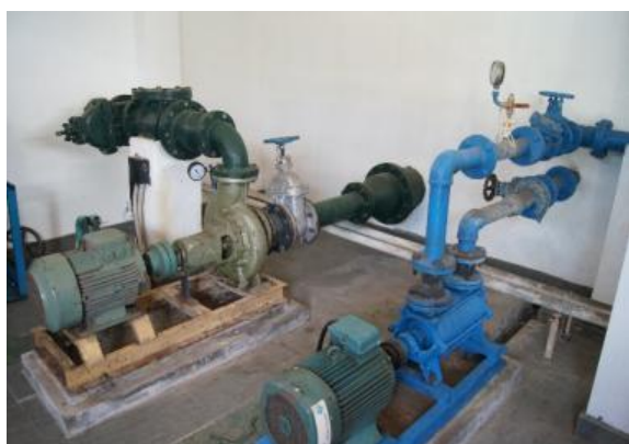
No.17 Chemical Injection Facilities in Brushn Water Treatment Plant
