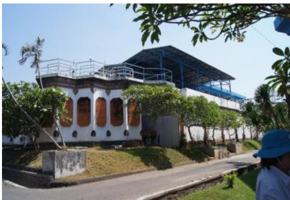
No.13 Brushn Water Treatment Plant (Denpasar)
