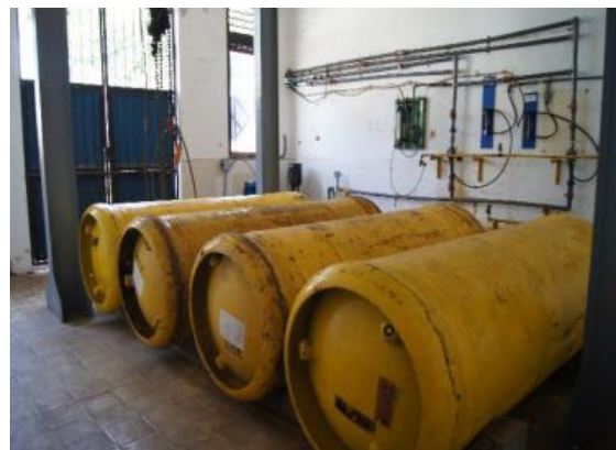
No.18 Chemical Injection Facilities in Brushn Water Treatment Plant
