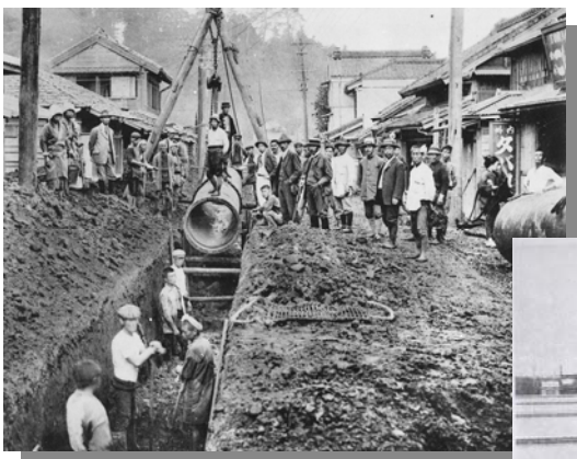
Pipe installation construction in Yokohama city (in the early 1910s)
