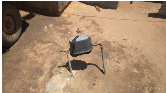
House connection installed in Nampula City
