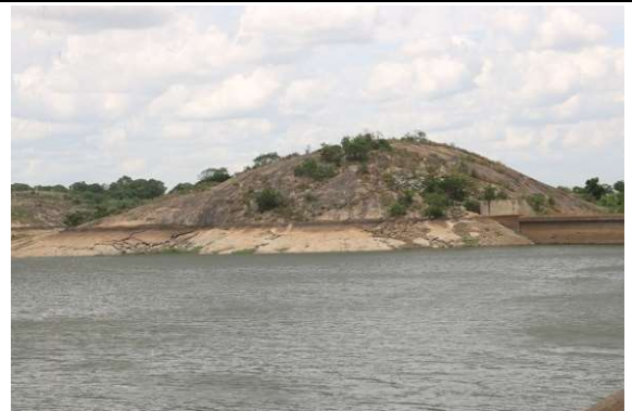
View of Nampula (Monapo) Dam (water level lowers during the dry season)
