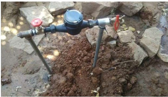
House connection installed in Nampula City
