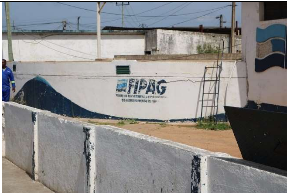
Pumping Station No. 3 (EB3) and reservoir
