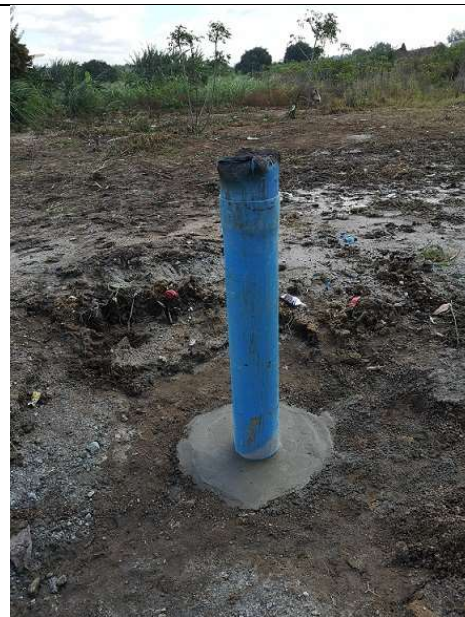
Figure 21 Existing Borehole (Pump Installation expected in 2021)
