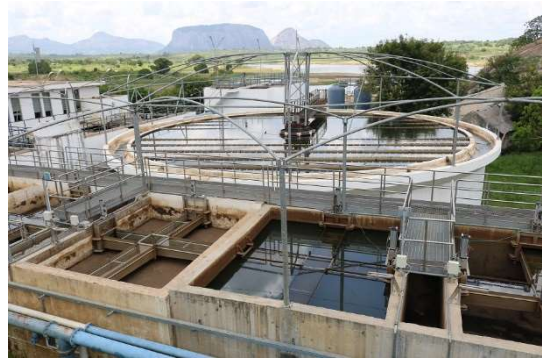
Water treatment plant at Nampula Dam
