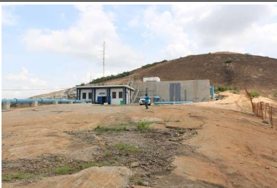
Distribution tank at Pumping Station No. 5 (EB5: 5000m 3 )
