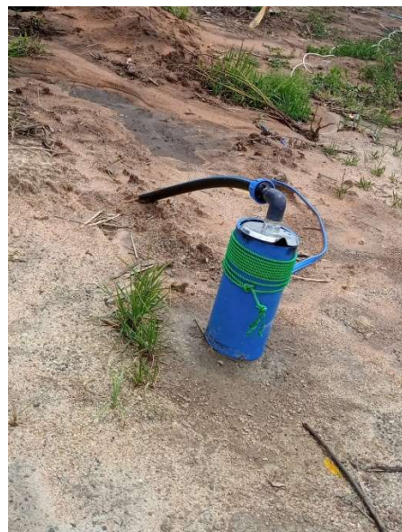
Borehole with pump constructed in 2020 in Namiteka area, south of Nampula city
