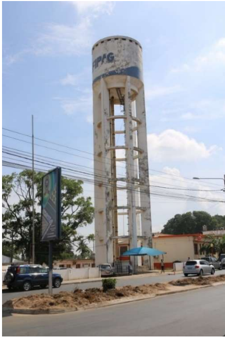
Elevated tank at Pumping Station No. 3
