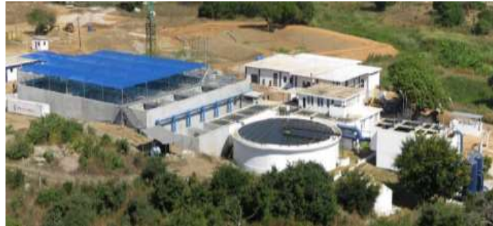
Figure 7 Nampula Water Treatment Facilities
