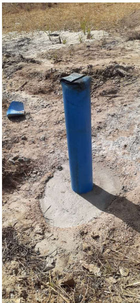
Borehole constructed in 2020 in Namiteka area, south of Nampula city
