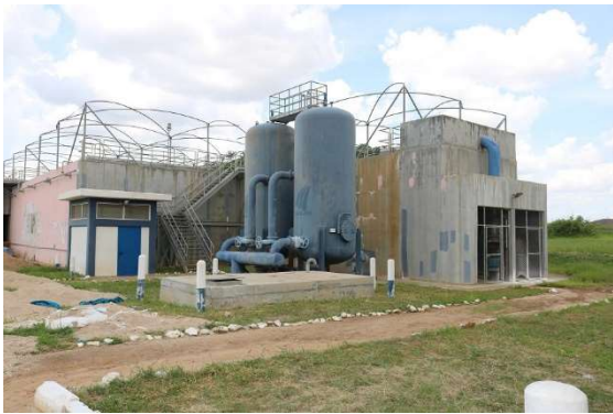
Water treatment plant at Nampula Dam
