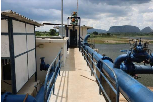
Water intake facility installed at Nampula Dam.
