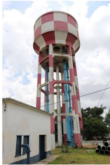
Elevated tank at Pumping Station No. 4
