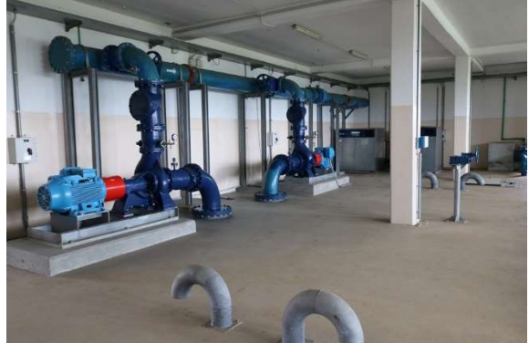
Interior of Pumping Station No. 1
