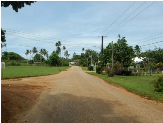
Photo-15: Road Condition at the Project Site
