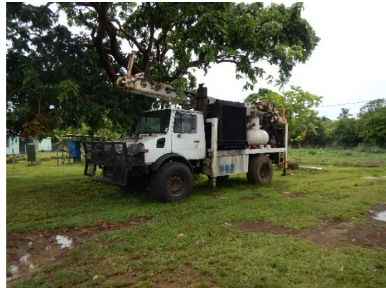
Photo-16: Drilling Rig for Well
