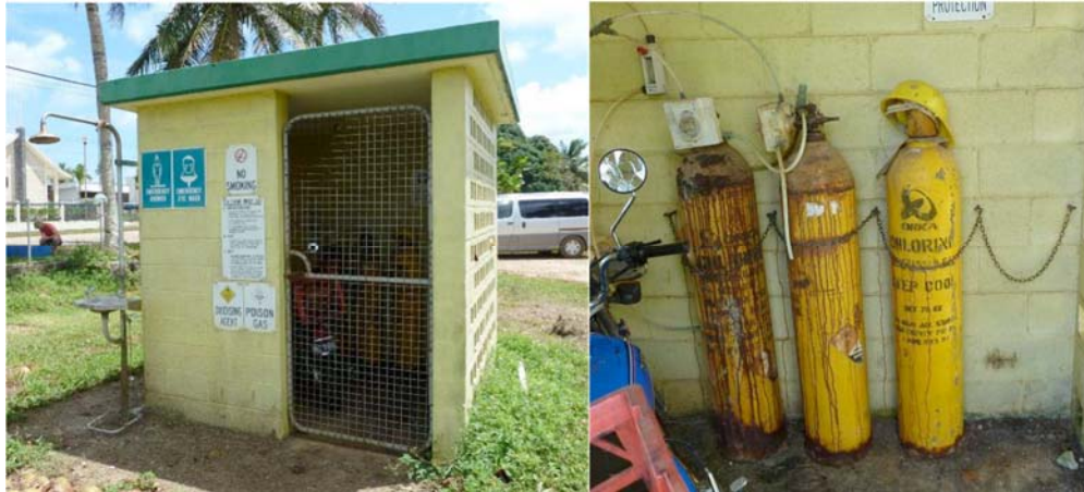
Photo 2.2 Chlorine Injection Unit that is not in Use
