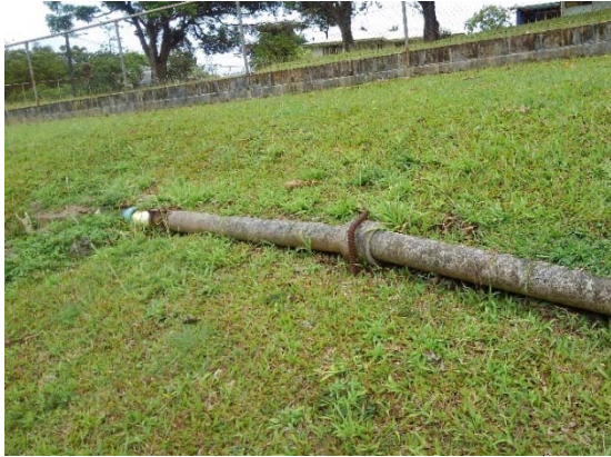
Photo-7: Asbestos Cement Pipe exposed on ground surface
