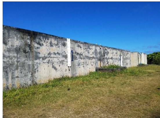
Photo-6: Existing Reservoir (Vava'u) RC structure of 1,400 m 3 (450 m 3 ×2, 500m 3 ×1). Efflorescence at some parts potentially caused by its deterioration was found on the wall surface.
