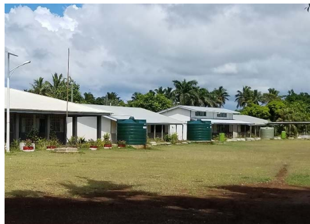
Photo 2.5 Rainwater Harvesting Facility set at School
