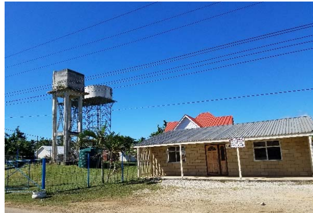
Photo 2.4 Water Supply Facility at Rural Areas
