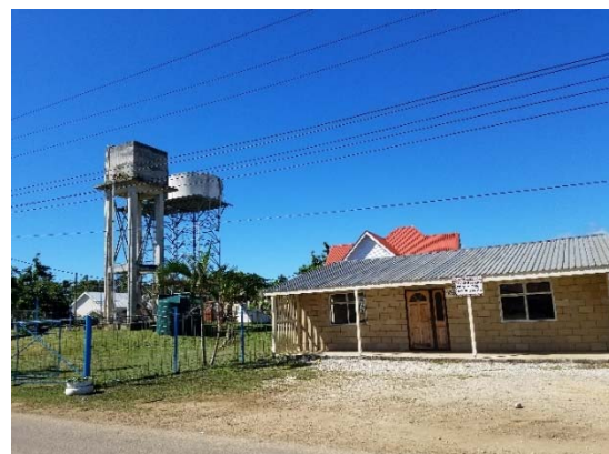
Photo-12: Water Supply Facilities at Rural Areas (1)
