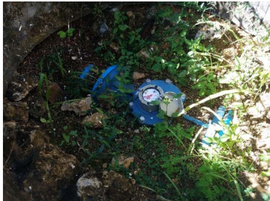
Photo-9: Flow Meter
