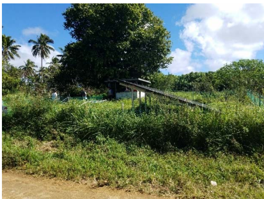
Photo-17: Solar Panel and Pump Unit that was procured by Japan ODA Assistance
