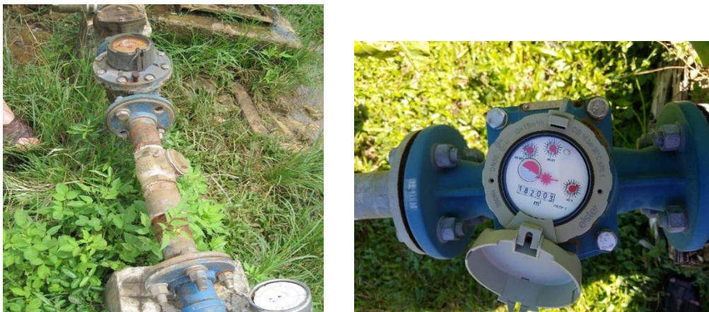
Photo 2.1 Malfunctional Flow Meter
