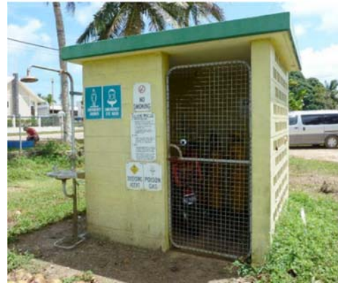
Photo-8: Chlorine Injection Unit (inside existing workshop)
