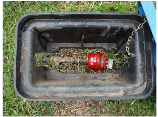
The current condition of water meter (house connection)
