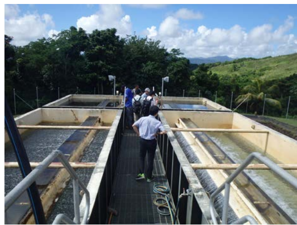
Northern Division (Labasa) Benau WTP; Clarifier
