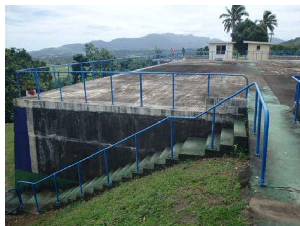
Northern Division (Labasa) Benau WTP; Benau Reservoir
