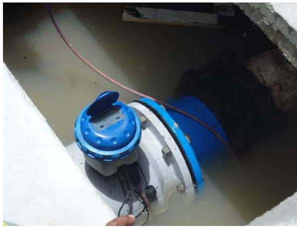
The current condition of DMA meter
