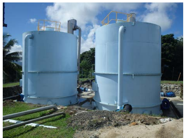
Northern Division (Labasa) Benau WTP; AVG filter
