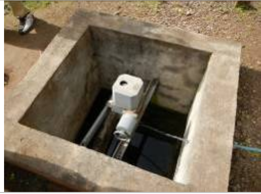
Water meter in Malkapur ESR, transmitting signal through exposed wire
