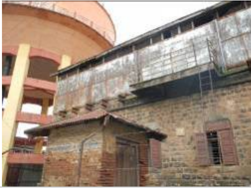
Office of MJP experts in Raviwar ESR site
