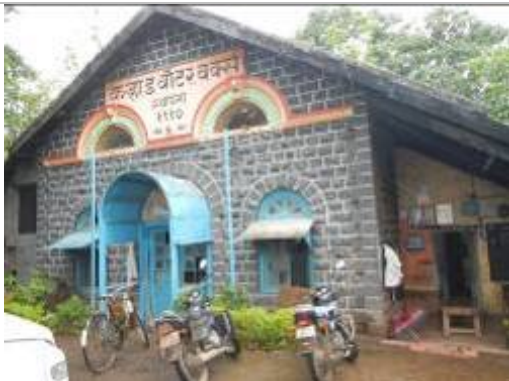
Office in the old WTP, to be demolished after construction of Super New WTP
