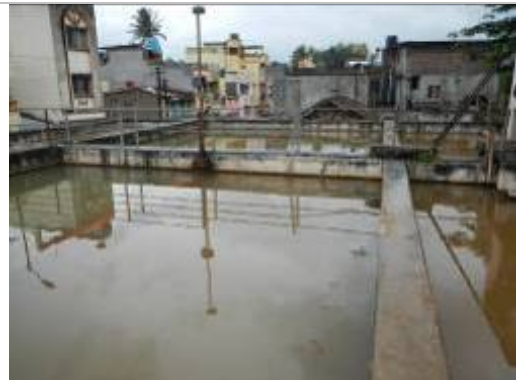
Coagulation tank in old WTP
