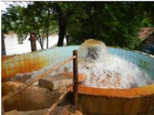
Lifted raw water at old WTP, with 150NTU
