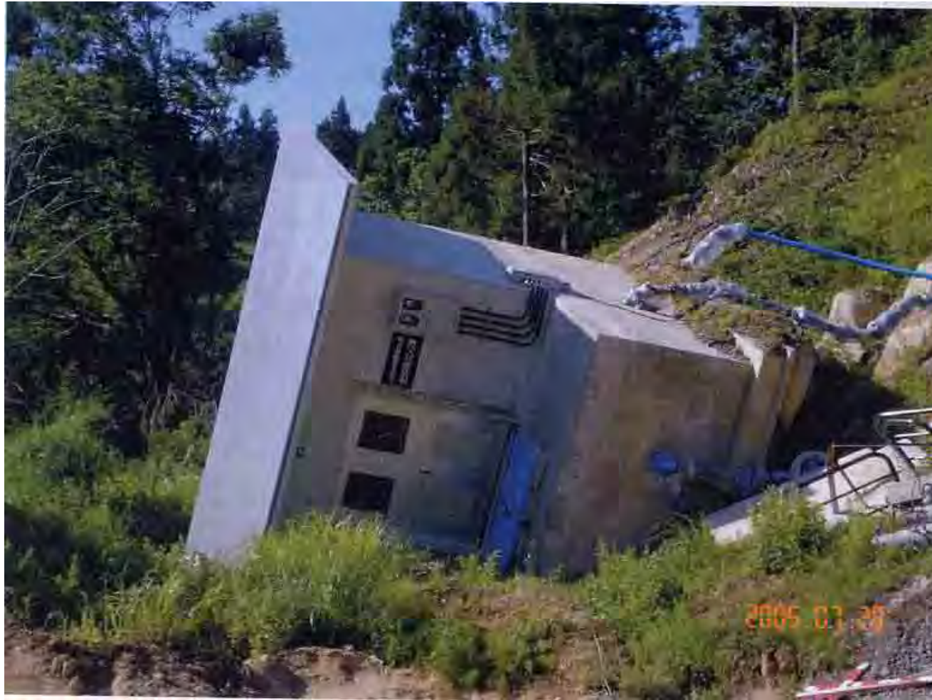
Collapse of an equipment shed
