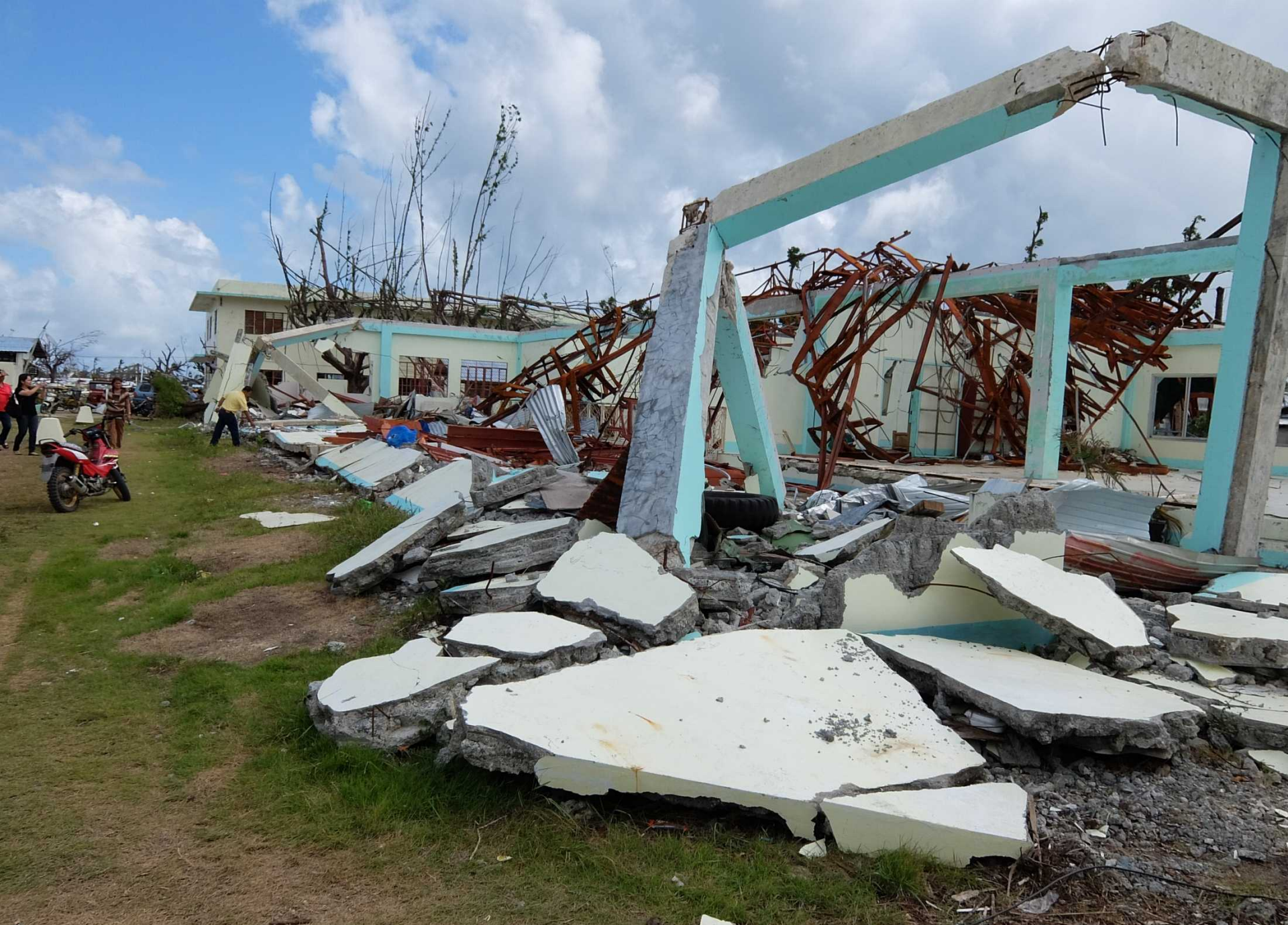
The Library of the Eastern Samar State University Guiuan was completely destroyed on 8 th November 2013 by the typhoon Yolanda.
