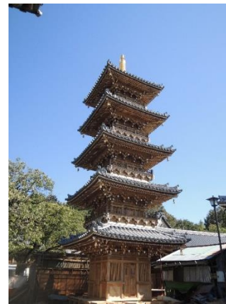
[拝島山本覺院五重塔新築工事]
