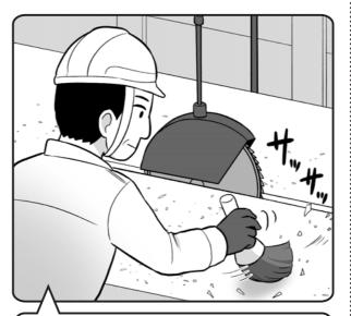
Turn off the machine when removing wood chips or sawdust.
