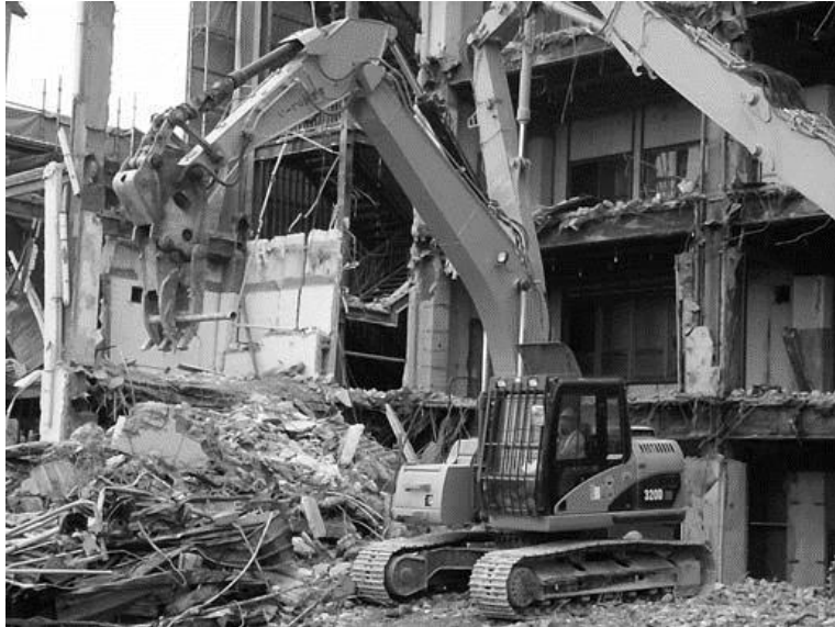
Larawan 1-6 Demolition Gripping Machine
