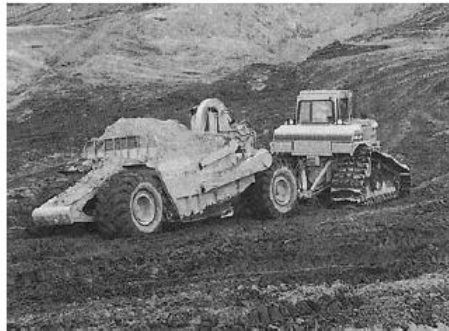
Litrato 6-6 Working status ng towed scraper
