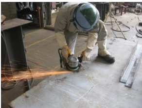
Grinder Polishing Work
