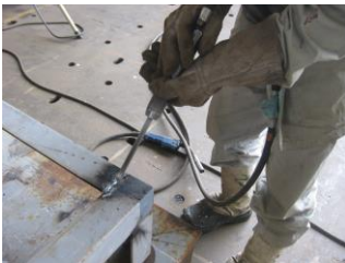
Chipper used for removing a welding slag
