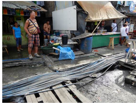
Service pipes connected to "Stub-out system". Mainly the pipes are on-ground. From the view of the pipes, it is called "spaghetti piping" and seen in Balangay water supply in the Philippines. (December 1, 2017)
