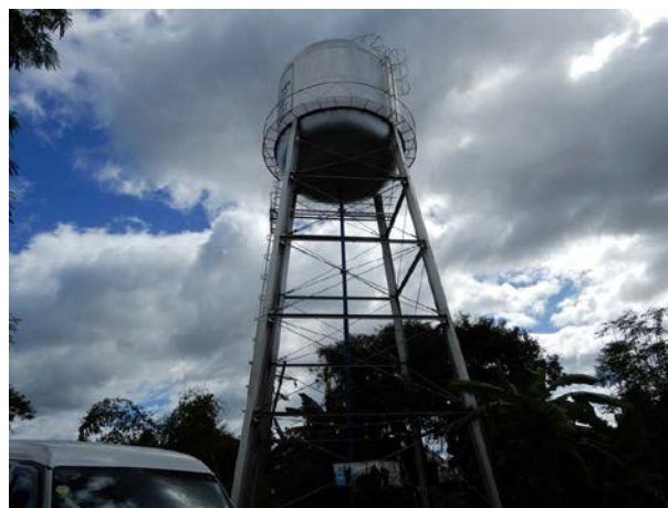
Figure 2-10. Elevated reservoir at San Jose Del Monte WD (COWD uses the same type)
