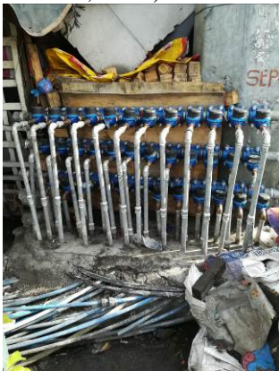
Faucet extraction system in Manila. This system is called "Stub-out" and used a lot in the Philippines. (December 1, 2017)
