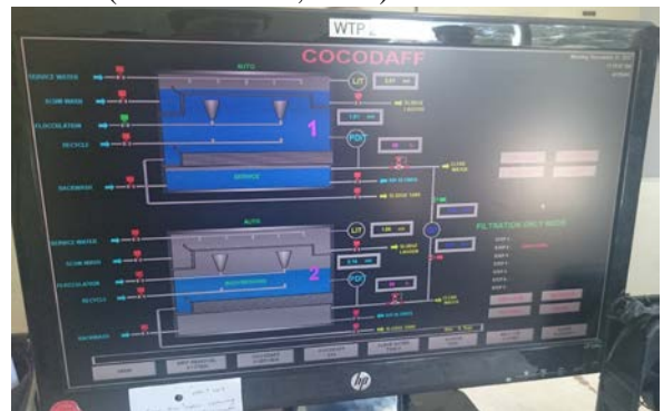
SCADA is ready at San Jose Del Monte Water District, which was supported by Yen loan project by Japan (November 27, 2017)
