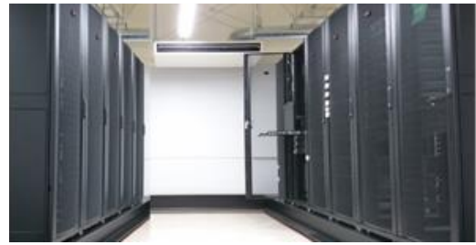
NCGG Data Server Room
