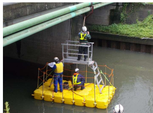
●浮き棧橋点検
