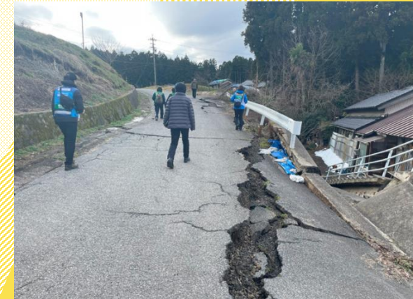
▲ Joint team including DPAT walked along cracked roads to visit isolated homes.
