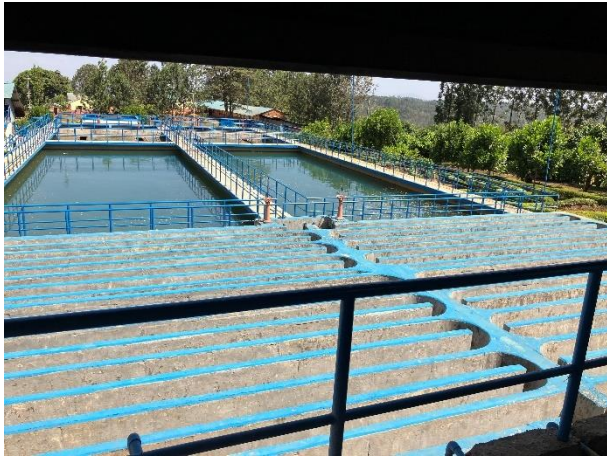
Photo 2-6 Flocculator and Sedimentation Basin
