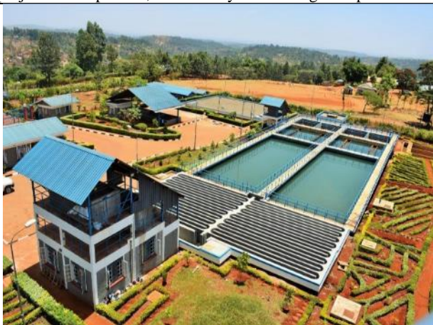
Photo 5: Kiawambeu Water Treatment Plant (WTP)
