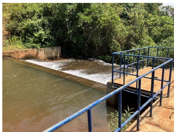
Photo 2-2 Intake Weir for Irrigation
