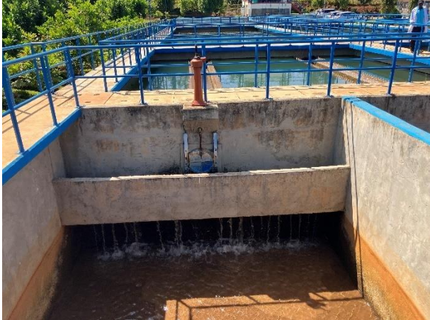
Photo 7: Rapid Sand Filter (Kiawambeu WTP)
