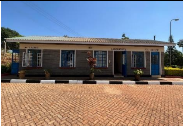
Photo 11: Management Office and Laboratory
