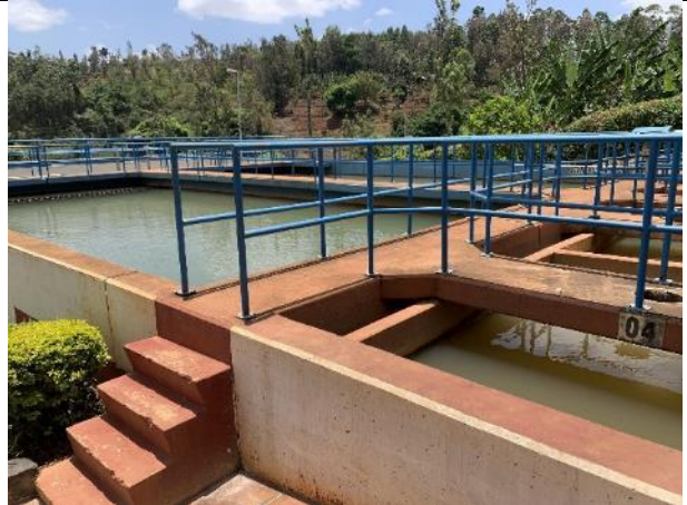
Photo 14: Kayahwe Water Treatment Plant (WTP)
