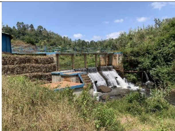
Photo 4: Water Intake Weir (Irati River)
