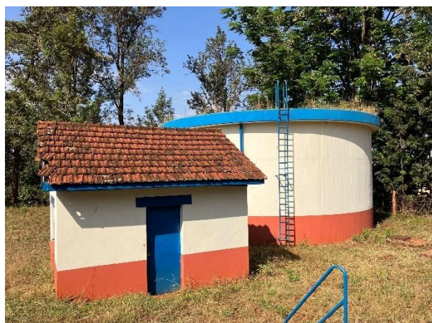
Photo 2-24 Maragi Reservoir (500 m 3 )
