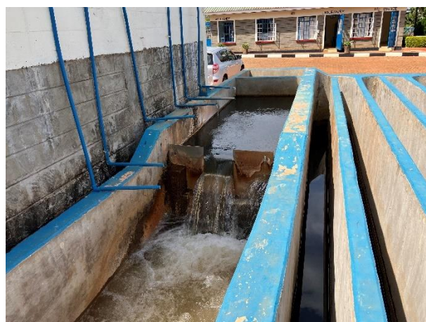
Photo 2-5 Receiving Well and Rapid Mixing
