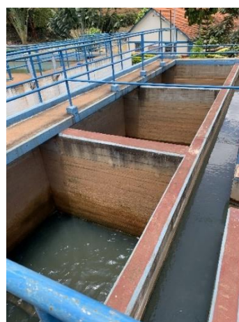
Photo 2-19 Rapid Sand Filter
