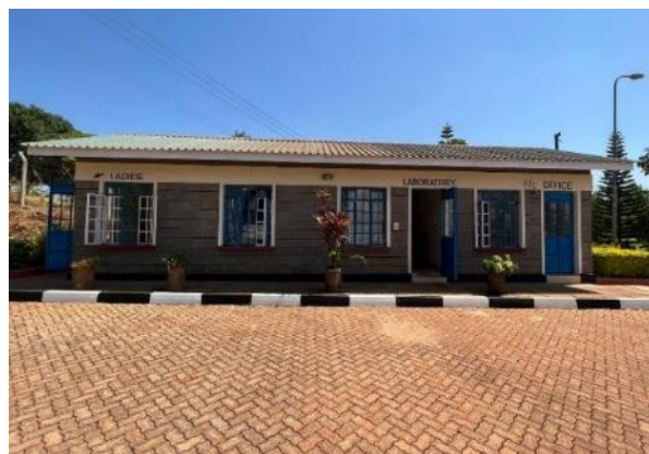
Photo 2-13 Management Office and Laboratory
