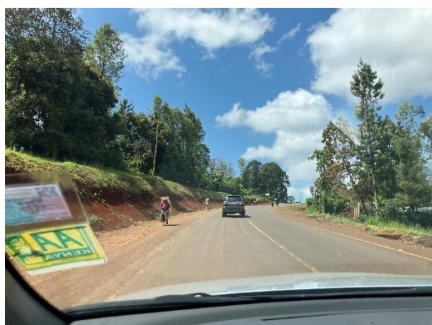
Photo 3-3 Road Condition for Pipeline Installation (Asphalt Paved)
