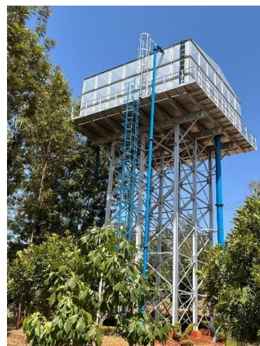
Photo 2-11 Elevated Tank (250m 3 )
