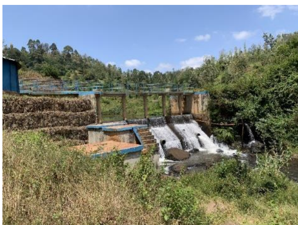
Photo 2-1 Irati Intake Weir
