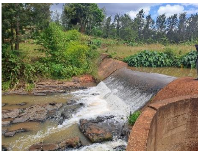
Photo 2-3 Kayahwe Intake Weir
