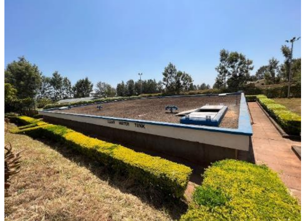
Photo 8: Clear Water Reservoir (Kiawambeu WTP)
