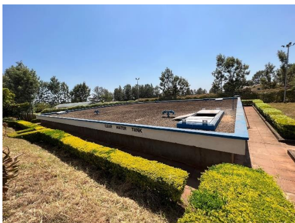
Photo 2-10 Clear Water Reservoir (2,000m 3 )
