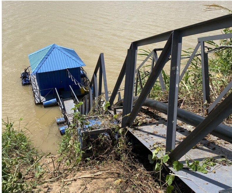
Figure 3: Water Intake at the Koh Dach Water Treatment Plant in Phnom Penh (provided by Kobelco Eco-Solutions Co., Ltd.)
