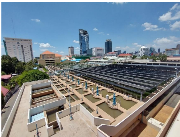
Figure 2: Solar power generation facilities at the Phum Prek Water Treatment Plant (Provided by MISTI)
