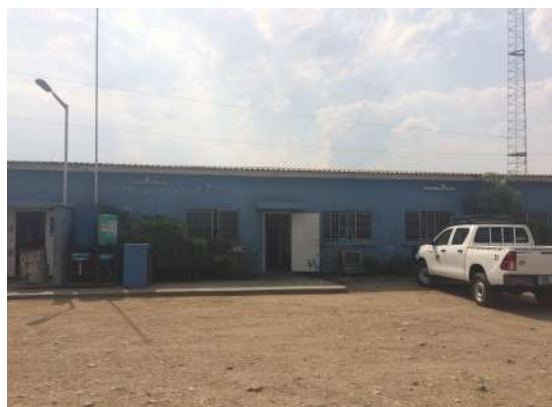
LWSC George office built with Japanese support
