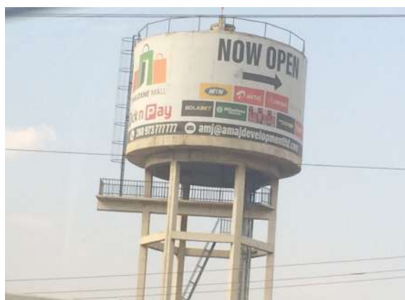
Concrete elevated water tank in George Area
