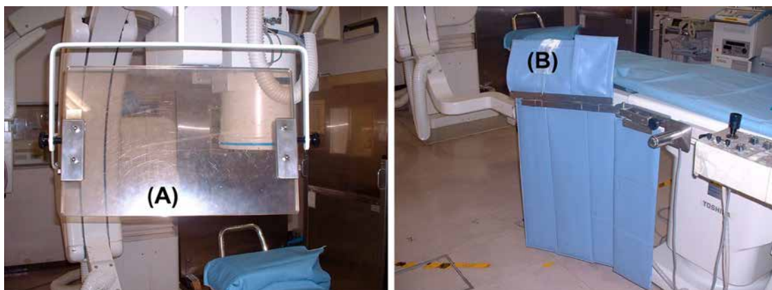
Fig. 2 Additional lead shielding devices. A Lead acrylic shields (0.8 mm-lead-equivalent) suspended from the ceiling. B Table side drapes (0.3 mm-lead-equivalent)
