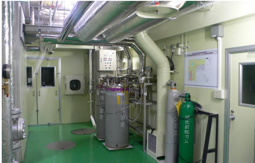
1. Entrance and Over view
