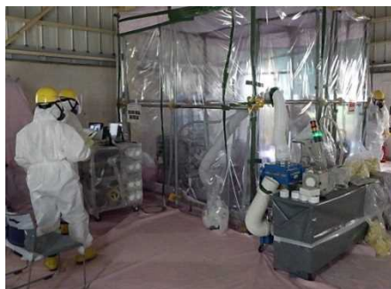
Photo 1: Appearance of analysis vessel installation (Red zone)
