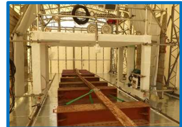
Remote-controlled cutting tool (wire saw)
