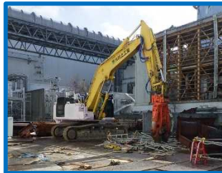
Remote-controlled heavy equipment (PC450)
