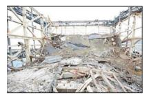
The collapsed roof of Unit 1 operating floor
