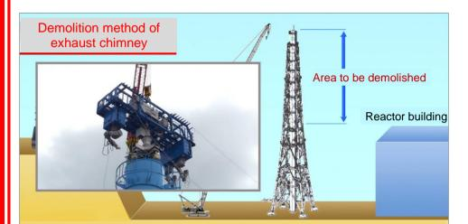
A crane is used to insert a demolition machine to the upper part of the chimney.
