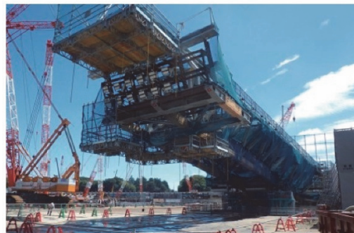
Assemble a full-scale mockup on the ground to check work procedures
