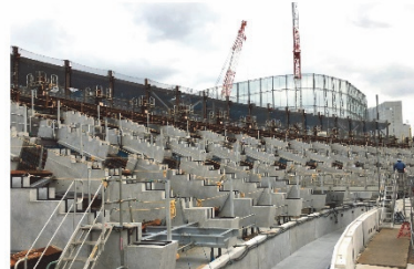
Floor slab receiving raker beam
