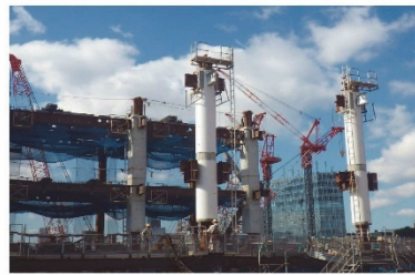
Outer SRC pillar
