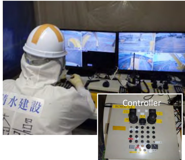
Operation of RCM from a remote room
