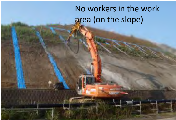
Shotcrete with a Robo-Shot
