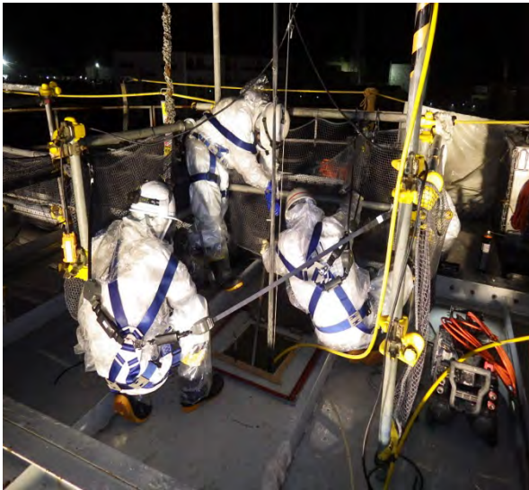
Wear safety harness in high places
