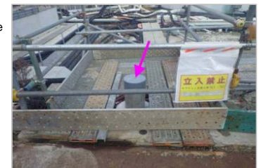
New sub-drain pit
