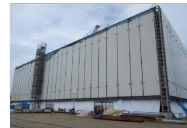
Building for expanded ALPS
