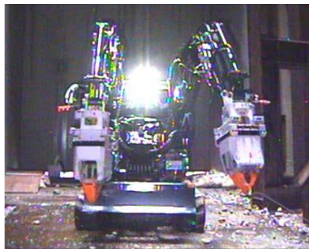
Remote-controlled removal of rubble in the R/B
