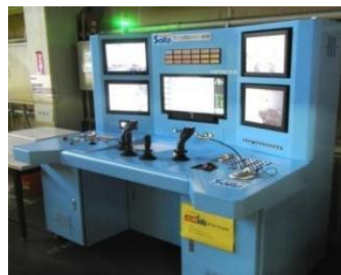
Important quake-proof building Operation panel
