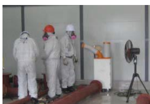
Using a spot cooler and large electric fan
