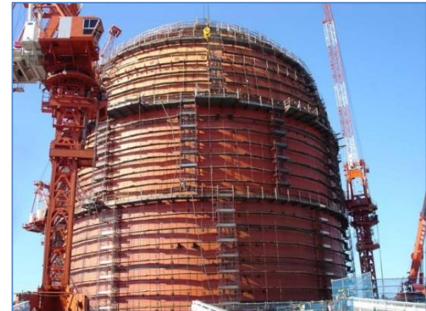
[原子炉格納容器の現地据付]
