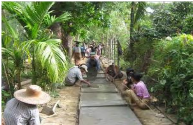
Workers from local communities pouring concrete to pave a village path, Myanmar
