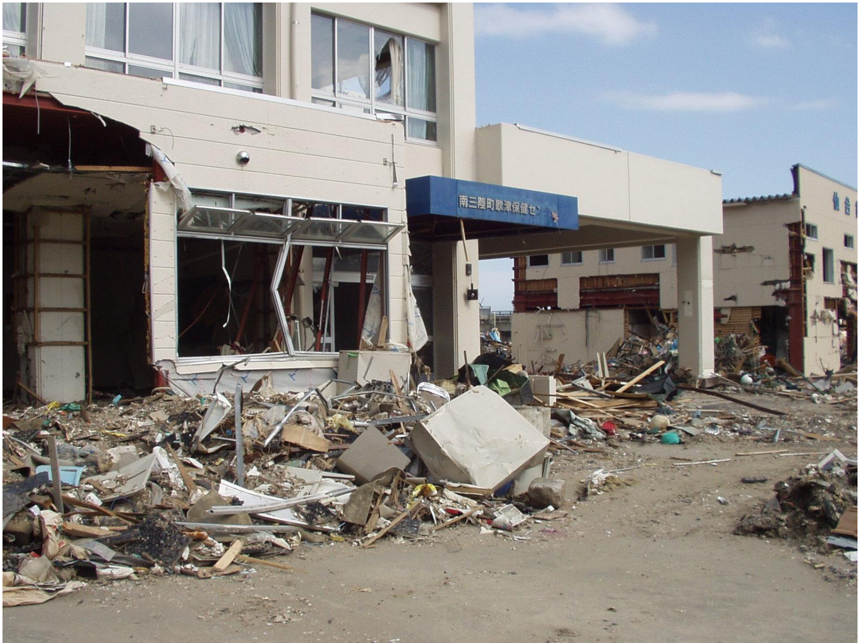
Health and Welfare Center in Minamisanriku Town
