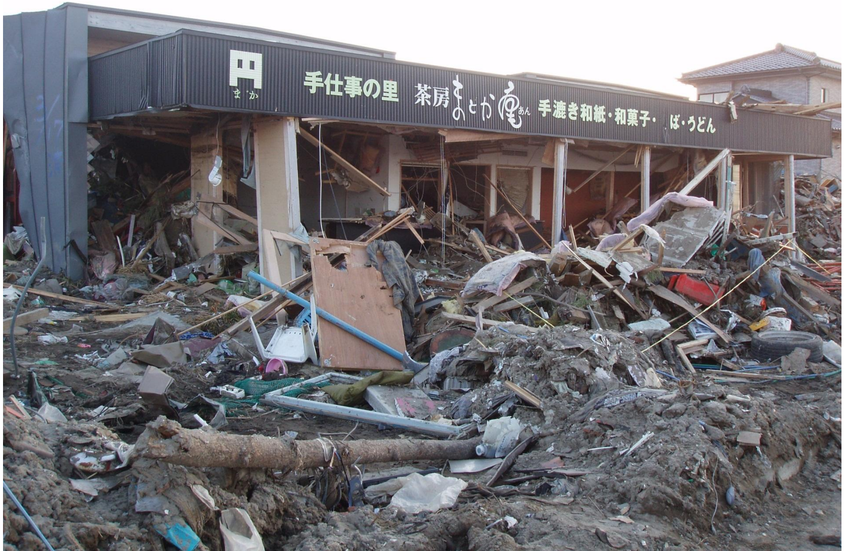
Madoka, facility completely destroyed by Tsunami
