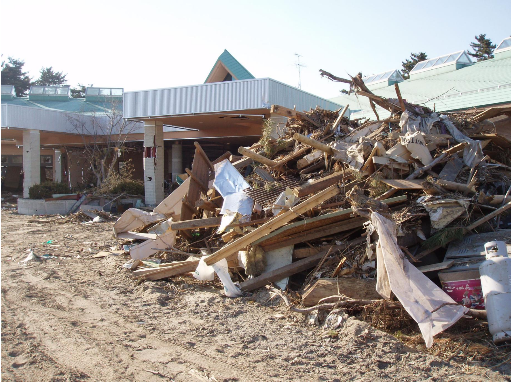
Rubato, completely destroyed facility
